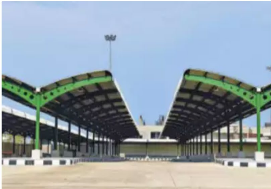
The Kilambakkam terminus, which is being constructed at ` 397 crore, was supposed to be inaugurated last year
